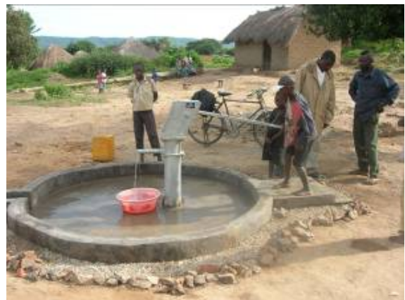
Installation of the water pump at Mpala
