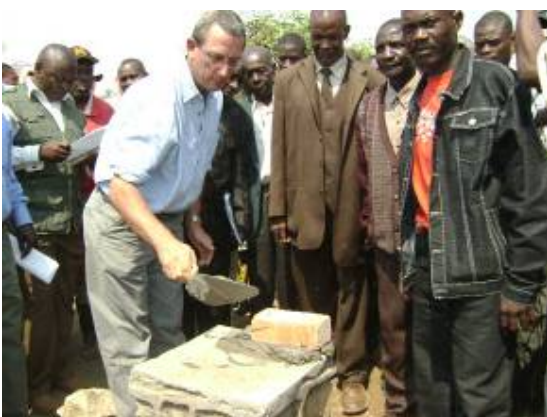
Official start of the construction of the Primary School in Muombe Mwewa, Kinsevere
