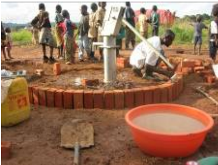
Building a water pump
