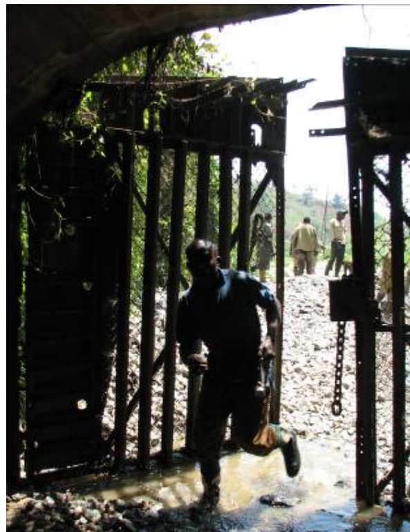
The challenge of closing the Addidi Mine, Mongbwalu where the miners are digging out the pillars that support the roof
