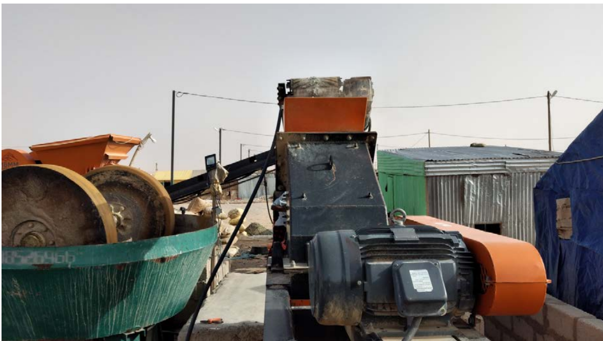
Picture 23: MBMM's turnkey ore processing system
