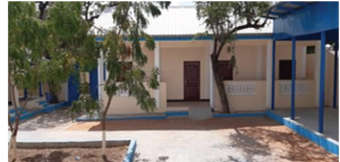
Wadajir district courthouse after rehabilitation. Photo credit: Pact Kenya.
